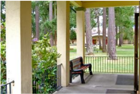
Patio Across from Exercise Hall
